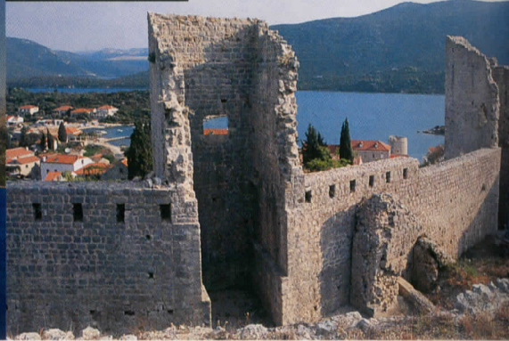
WONDER WALL: Feel inspired by the legends that surround the walls of Ston
